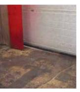
Roll-up doors should be fitted with a flexible bottom "seal" and T extensions to fit rail tracks.
