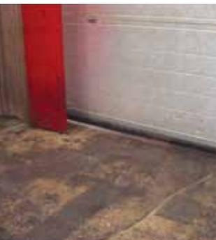
Waste skips should be placed on a concrete pad to prevent rats burrowing underneath and be situated on rails of a height that will allow for thorough cleaning below. The concrete should be capable of carrying rainwater and run-off from cleaning to a drain.
